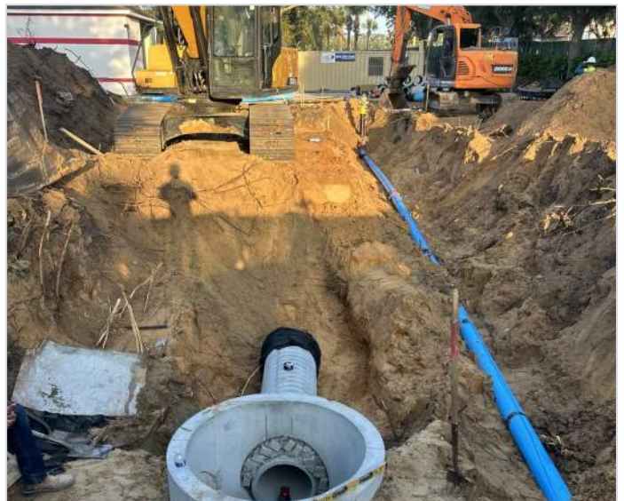
STORM DRAINAGE & UTILITIES
